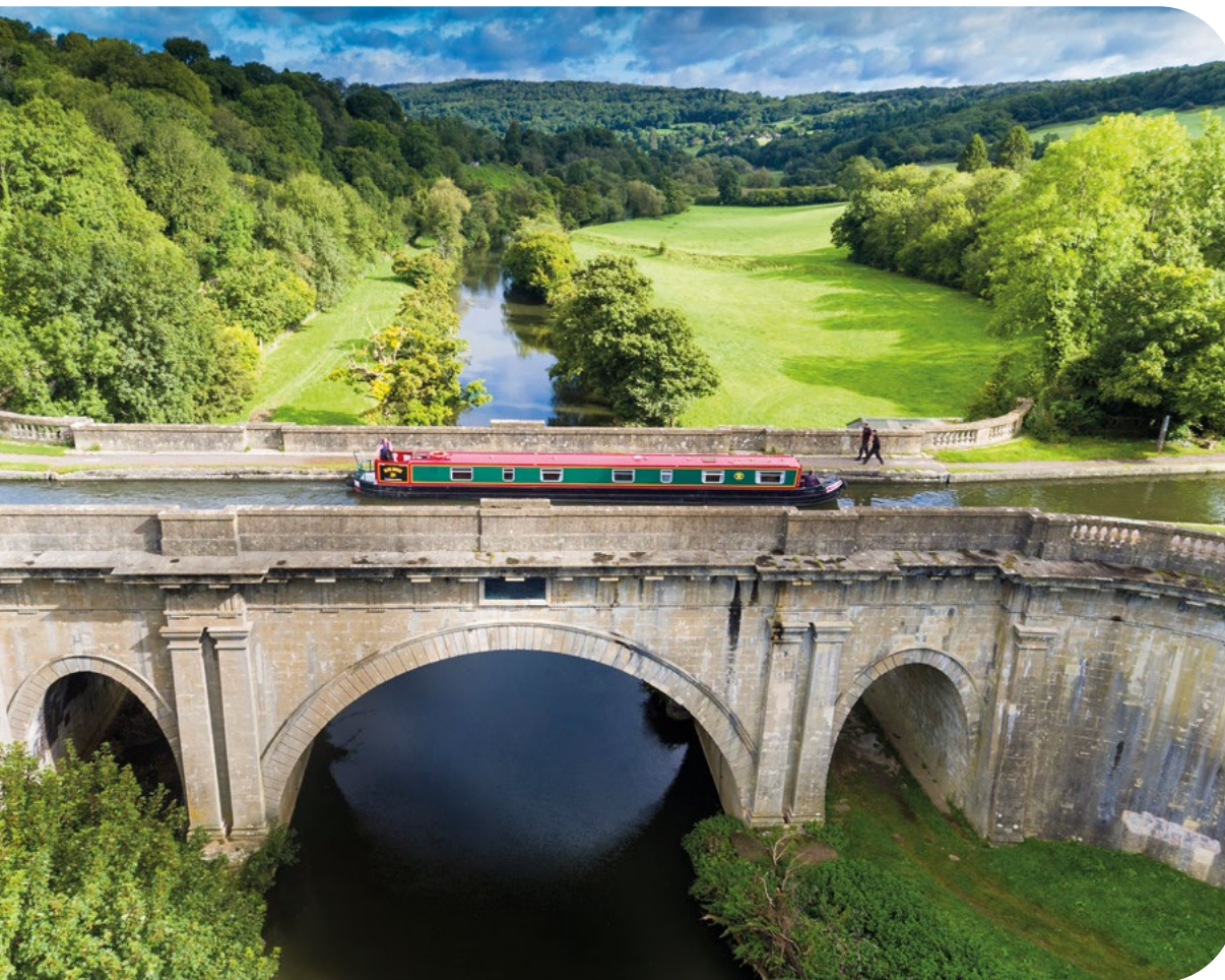
Left: Dundas Aqueduct, Kennet & Avon Canal
