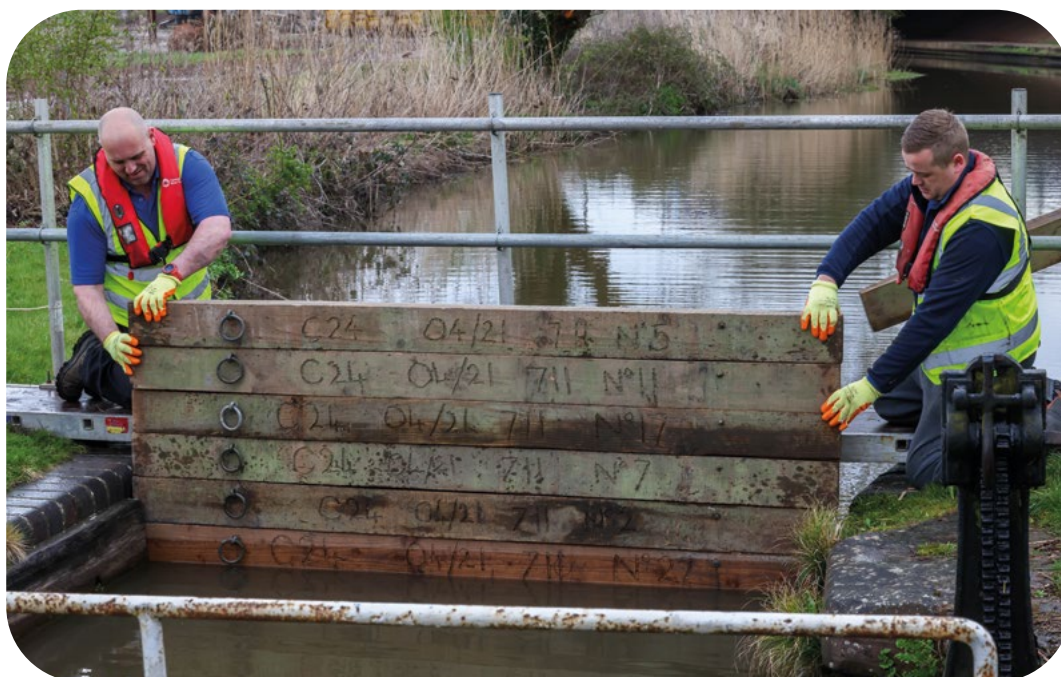
Left: Offerton, Worcester & Birmingham Canal
